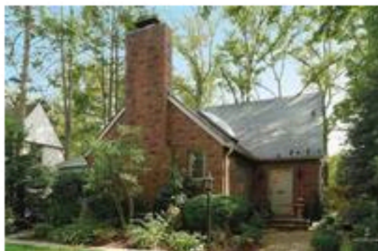
BEFORE: The front of the house prior to renovation.
