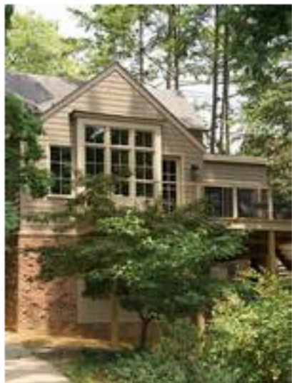
The renovated house from the back.
